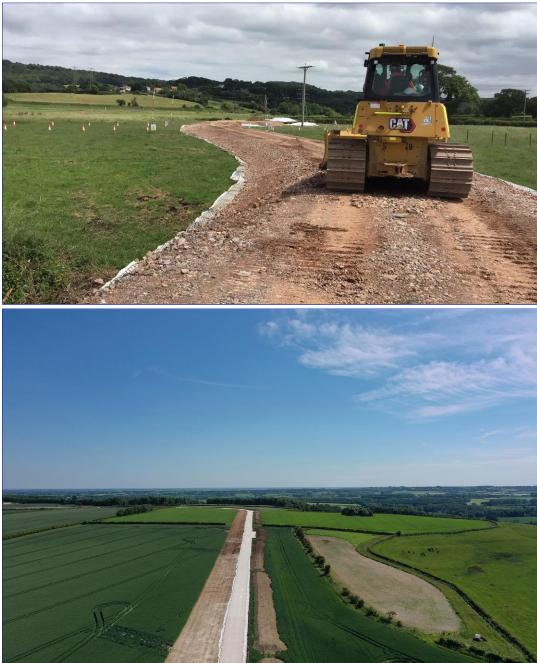
Figure 6.1: Typical temporary access roads constructed with stone
